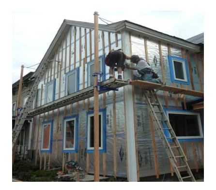
Rainscreen w/ 1x3 strapping provides <sup>3</sup>/<sub>4</sub>" drainage and ventilation gap
