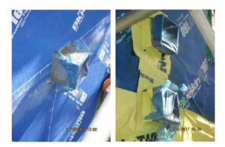
Central vs. Unitized: Wall penetrations from in-unit ERVs
