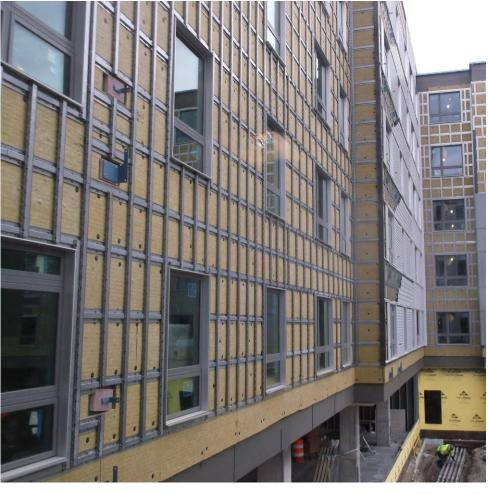
Finch Cambridge - Cascadia Clips The Loop – Knight Wall System Both provide rainscreen and thermally broken siding connections
