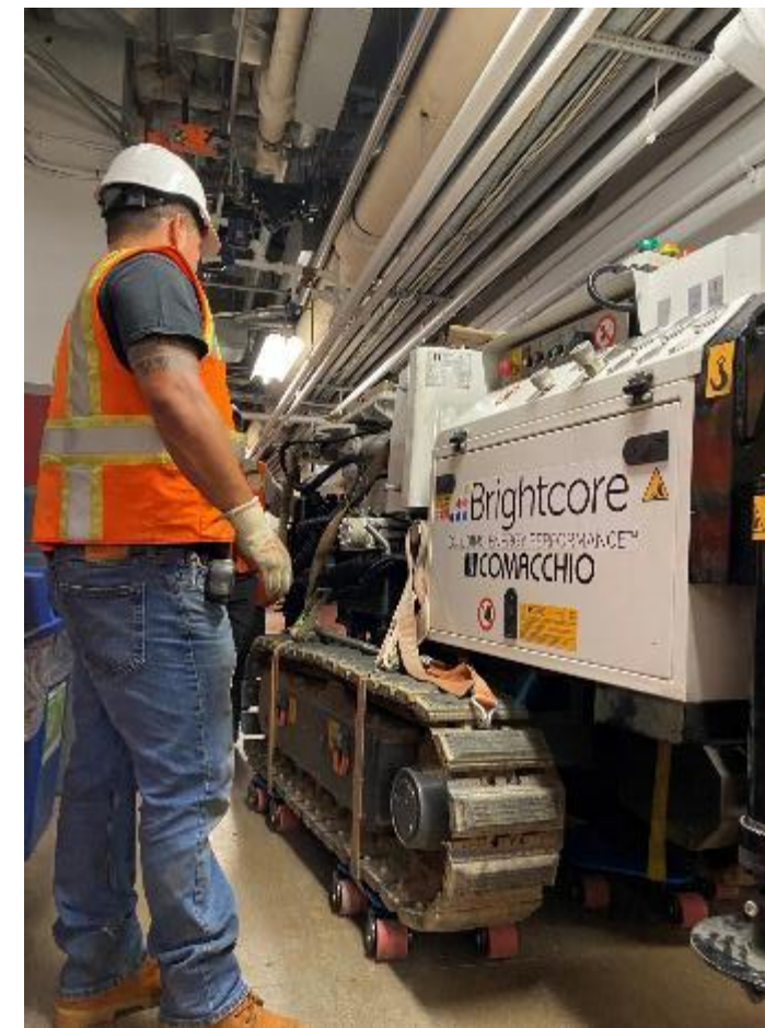
Brightcore's custom mini-rig entering and drilling from within the basement of a century-old co-op in Manhattan
