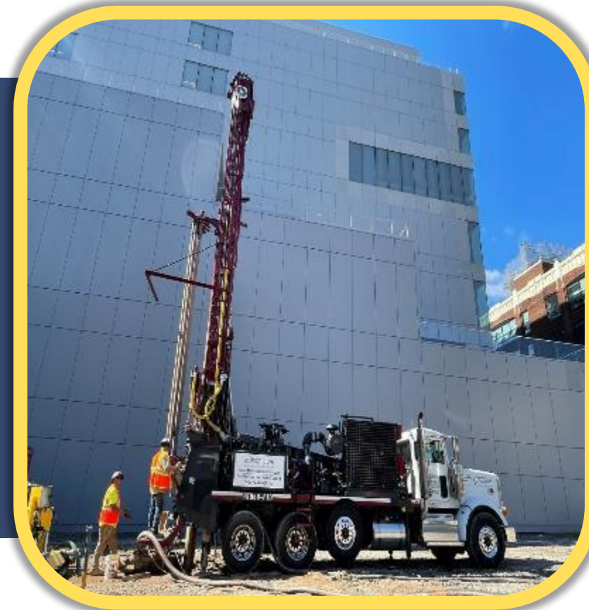
TRUCK MOUNTED RIG
