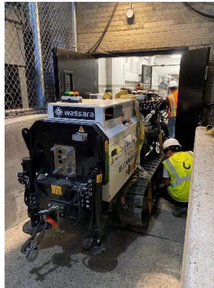
Brightcore's custom mini-rig entering and drilling from within the basement of a century-old co-op in Manhattan
